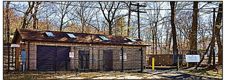
North Broadway Pump Station - North Castle, NY
